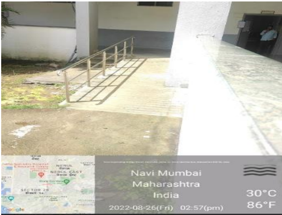
Fig. Ramp for physically disabled person
